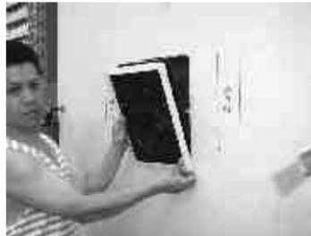
**4**) Align the speaker in position, and tighten the screws evenly to secure the unit.
